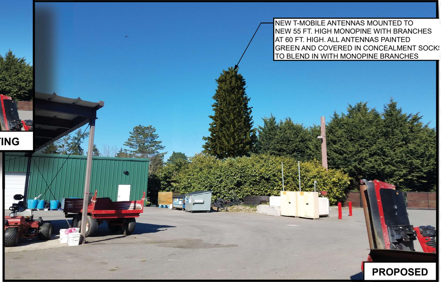
NEW T-MOBILE ANTENNAS MOUNTED TO NEW 55 FT. HIGH MONOPINE WITH BRANCHES AT 60 FT. HIGH. ALL ANTENNAS PAINTED GREEN AND COVERED IN CONCEALMENT SOCKS TO BLEND IN WITH MONOPINE BRANCHES
